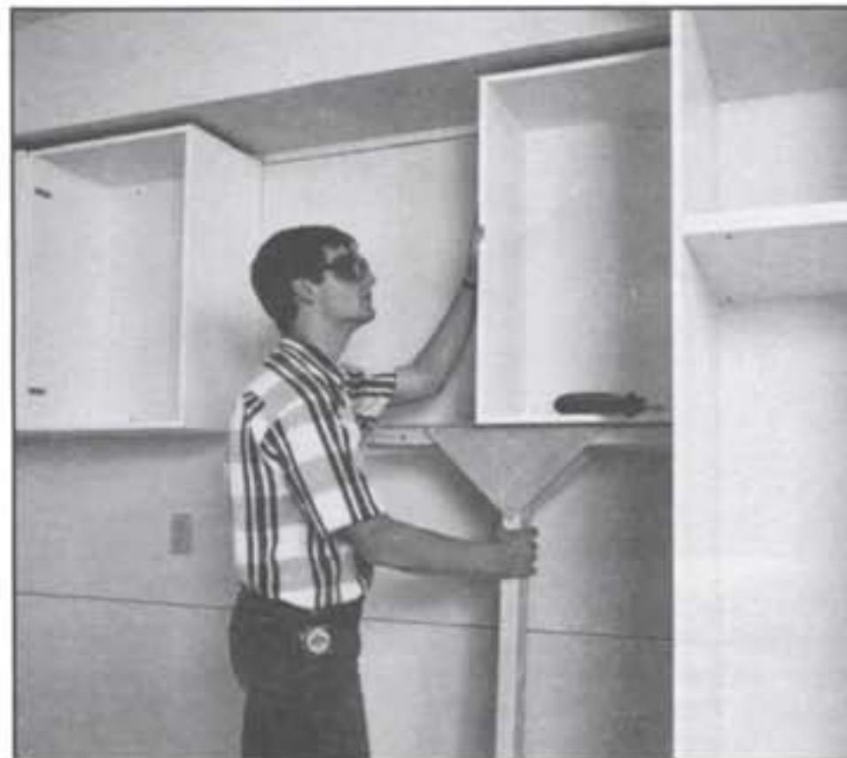
Use the T-Bar method to install wall cabinets.
